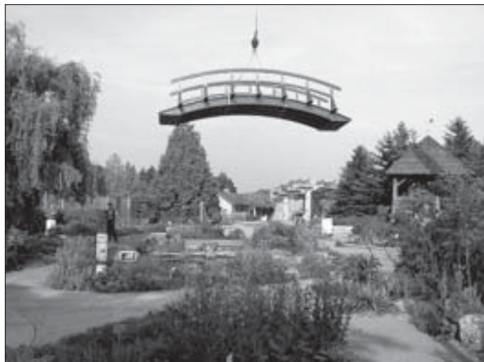
The Michigan 4-H Children's Garden pond and Monet Bridge underwent major renovations earlier this summer. The pond liner needed to be replaced, so the Monet Bridge was lifted out of place and stored for two weeks in the parking lot. 4-H Children's Garden student interns cleaned and stripped old paint from the bridge, rescued the turtles and fish from the pond and cared for the animals during the renovations.
